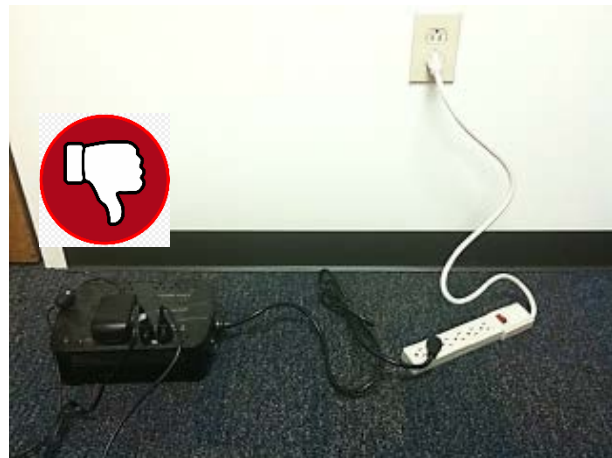
Power strips may not be plugged before or after an uninterruptable power supply (UPS).
